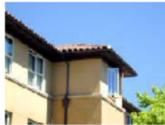
Kimball Hall roof overhang, 1991 (BAR)
