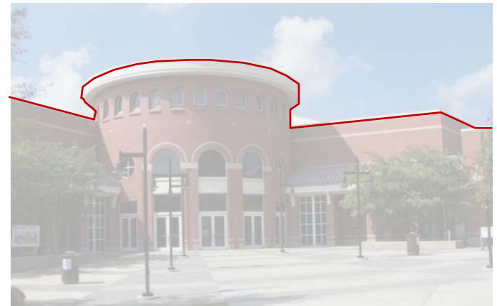
Flat roof with parapet
