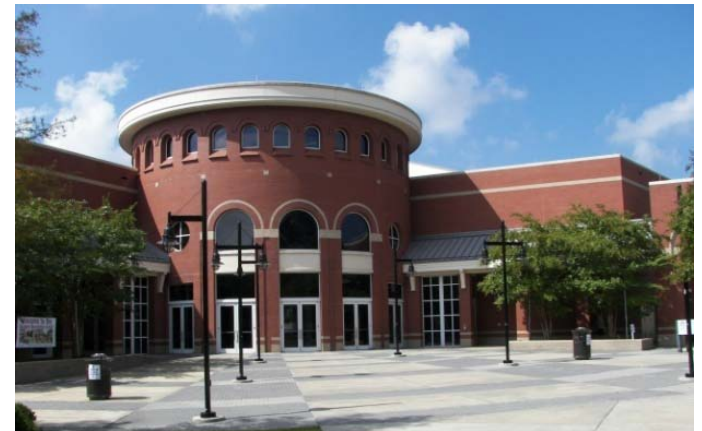
Flat roof with parapet
