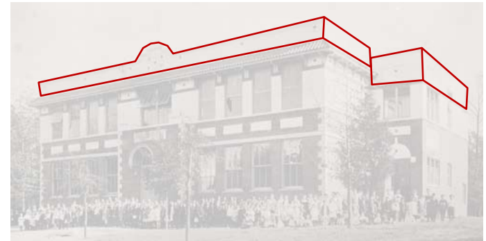
Flat roof with false front
