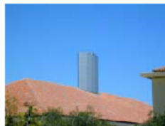
Moore Building roof stack, 2000 (Pei Cobb Freed and Partners)
