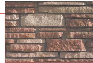
A close-up detail photo of a typical sandstone wall.
