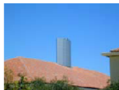
Moore Building roof stack, 2000 (Pel Cobb Freed and Partners)
