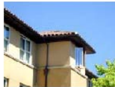
Kimball Hall roof overhang, 1991 (BAR)
