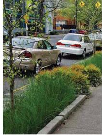
An inlet from the curb allows water to enter the infiltration planter.
