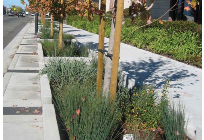
Landscape planters also function as stormwater infiltration areas.
