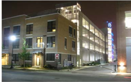
Ohio State University, wrapped parking deck
