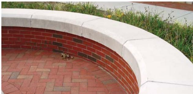
Seatwalls should be capped with limestone or cast stone.
