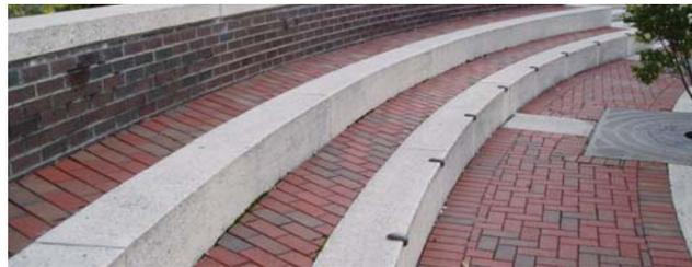
The stepped wall detail in Sonic Plaza uses a textured concrete cap.
