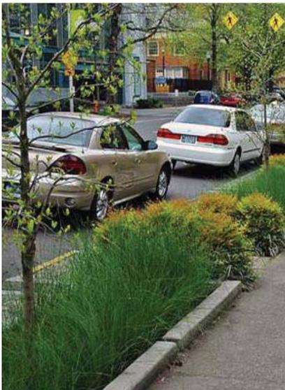
An inlet from the curb allows water to enter the infiltration planter.
